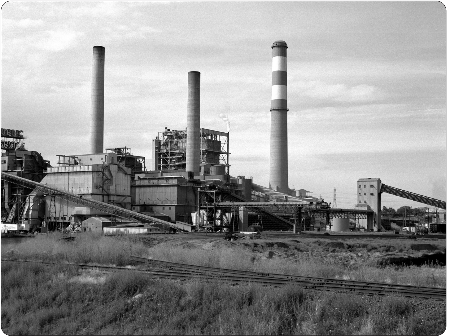
A coal power plant
