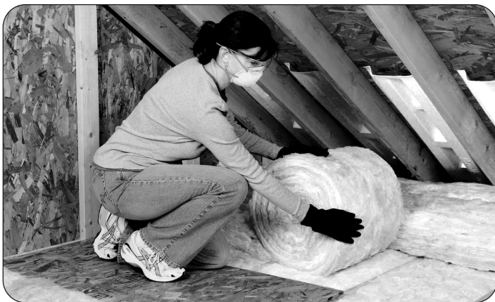
Image courtesy of Owens Corning
