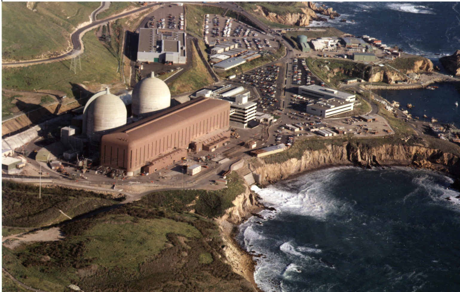
Diablo Canyon Nuclear Power Plant in California.
