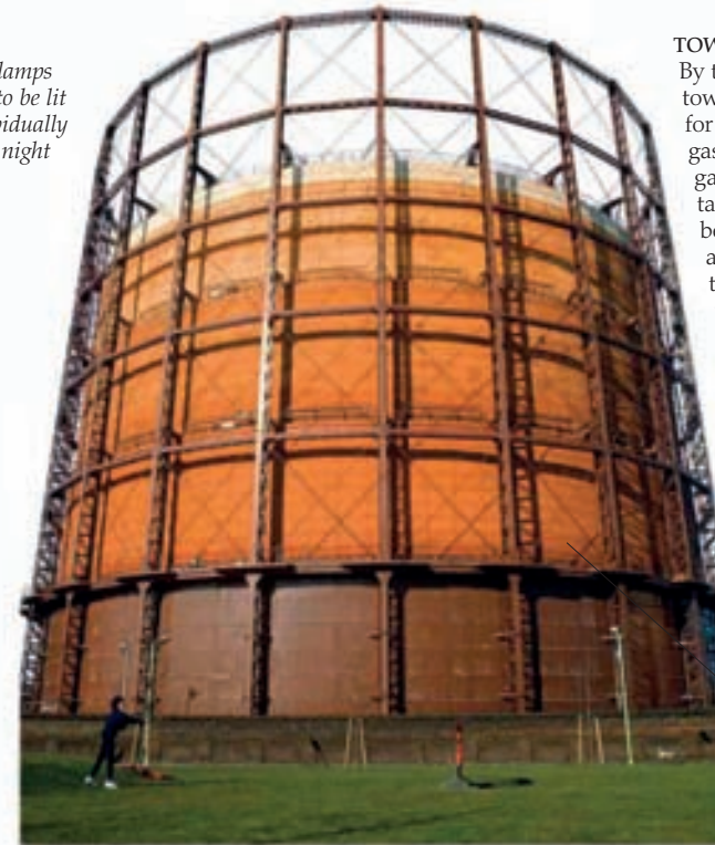
Gasometers sank into the ground as the level of gas inside went down
