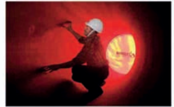
Worker inspecting a natural gas pipe, Russia
