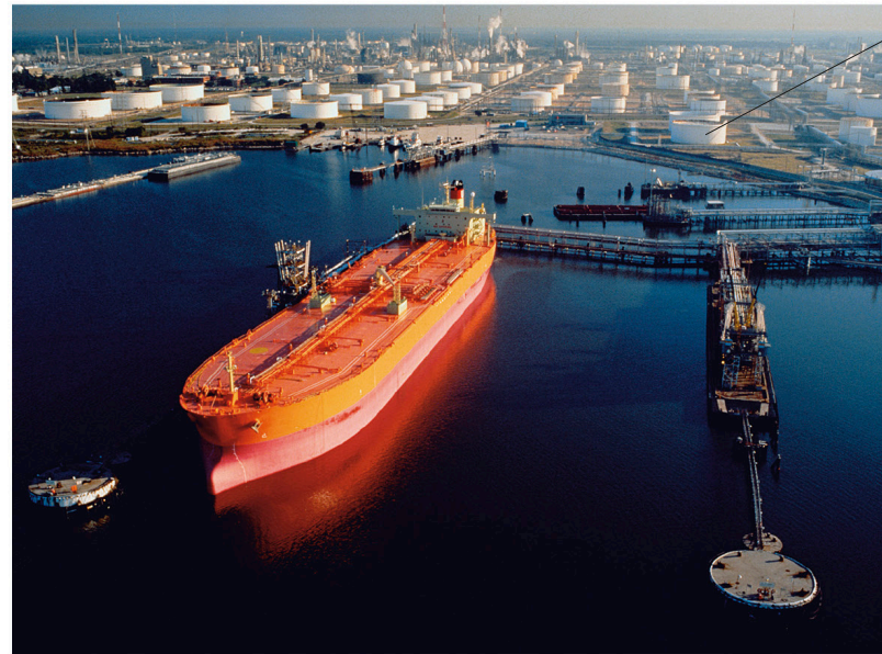
Onshore storage tanks
