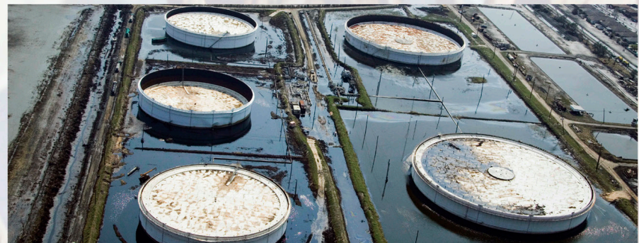
A flooded oil installation in the US hit by Hurricane Katrina in 2005
